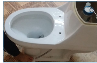
Fig. 4 Application of bowl-rotatable blade on a ceramic seat
